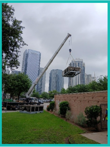
A crane at work replacing the air conditioning unit for the second floor of the Education Building.
